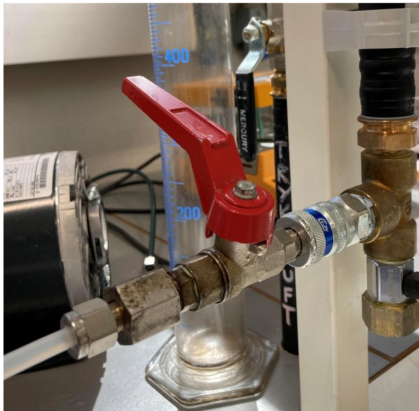
Figure 59 Air Source at the Laboratory
