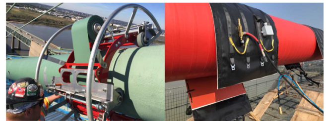
Figure 18: Pictures of the manual application process of the CableGuard system and heat sealing (Mathey, 2020).
