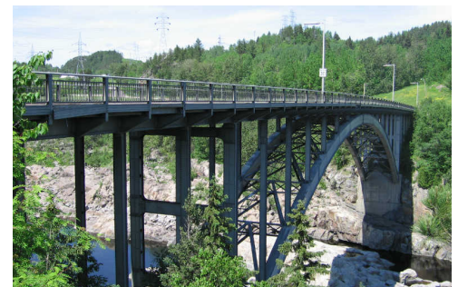
Figure 3: Side view of Arvida bridge (Potvin, 2006).
