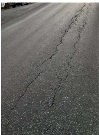
Figur 28: Langsgående sprekker
