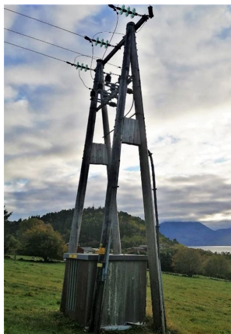
Figur 6: Masttransformator
