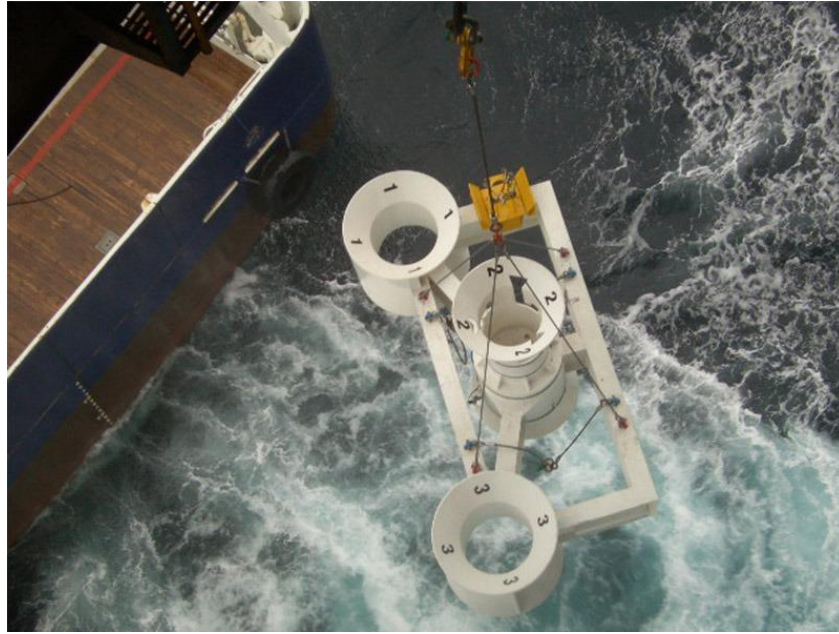
Figure 5.2 A subsea drilling template adopted from (Aquaterra, 2020)
