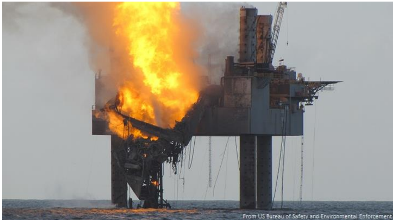
Figure 5.3 A natural gas well blowout in the Gulf of Mexico (Snow, 2015)
