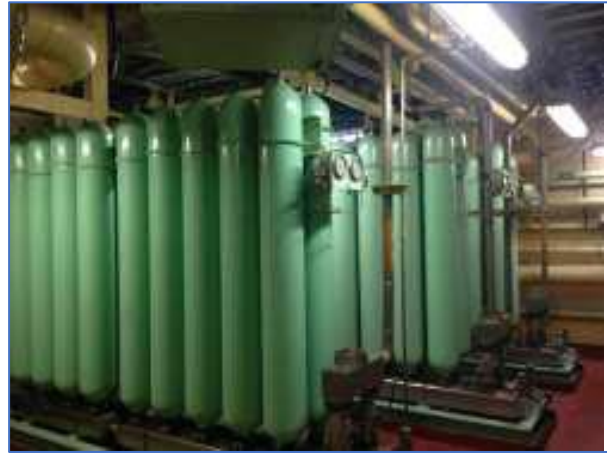
Figure 13: 15-gallon hydraulic bottles (Kazbekov)
