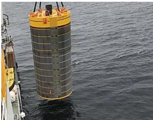
Figure 4: CAN about to be installed in the Barents Sea in 2018 (Neodrill AS 2020)
