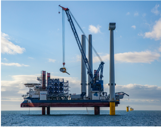
(a) Lift-off from vessel deck
