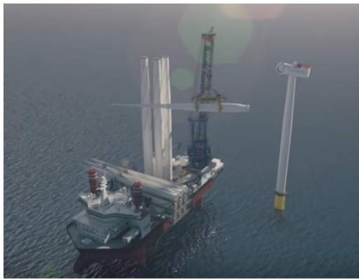
(b) Lift blade to hub-height
