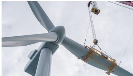
(e) Mating phase off blade-root and hub
