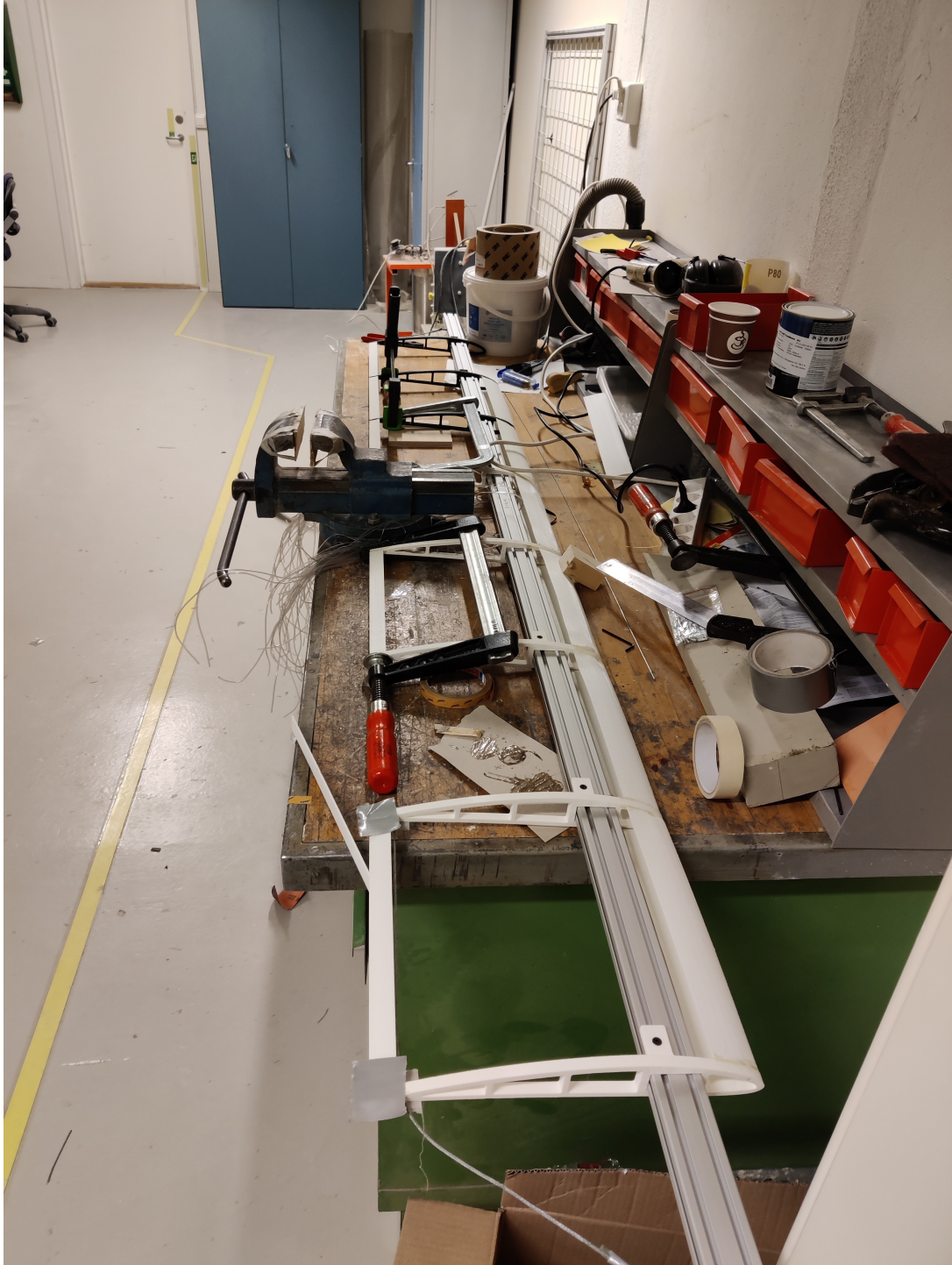
Figure 22: Mounting of the leading edge and trailing edge structure
