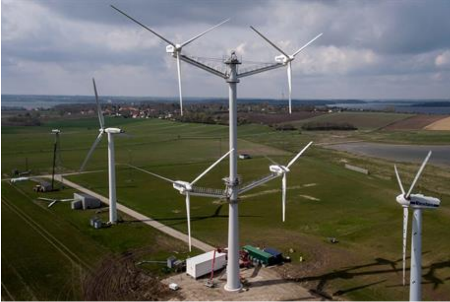
Figure 2.3: The Vestas Multi-rotor wind turbine[21]
