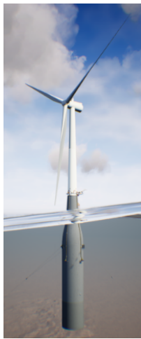
(a) SPAR monopile (A. Equinor 2019)
