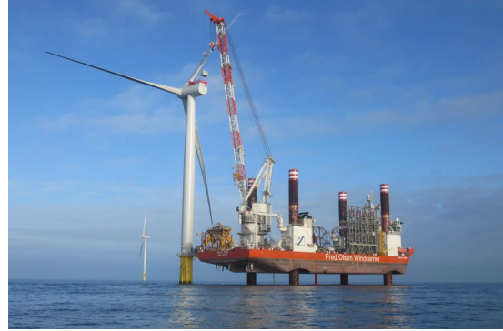
Figure 3.13: Jack-up crane vessel in operation. [19]
