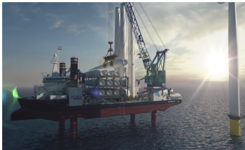
Figure 3.4: Step 2: Lifting the blade to hub height. [17]
