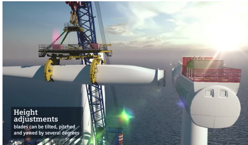
Figure 3.5: Step 3: The blade root approaches the hub. [17]
