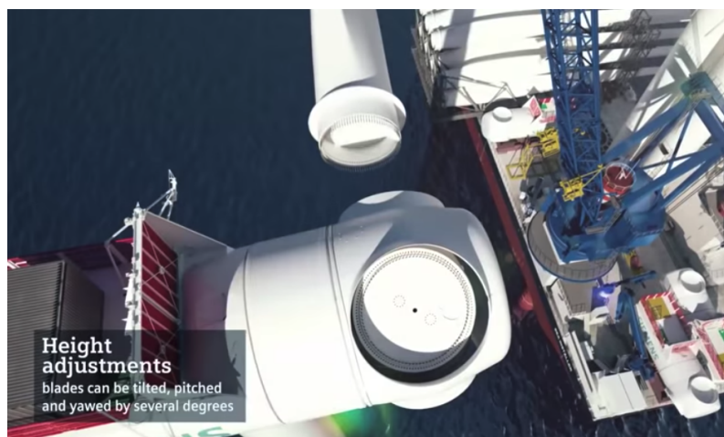
Figure 3.6: Step 4: Monitor the blade root motion. [17]
