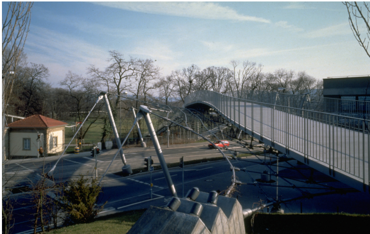
Figure 5.2: Lodz Footbridge: cable net
