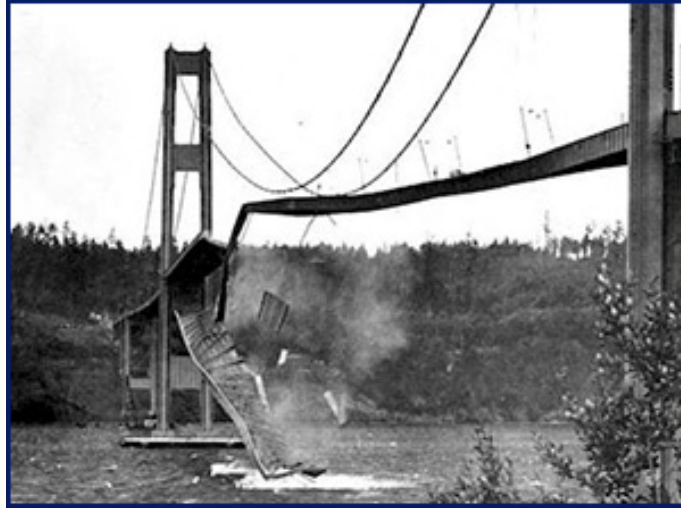
Figure 3.4: The collapse of Tacoma Narrows Bridge. [12]
