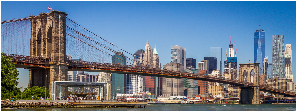
Figure 3.2: Brooklyn Bridge. Built in 1883. [28]
