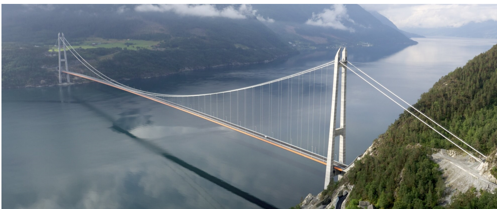
Figure 3.8: Hardanger Bridge. Built in 2013. [22]
