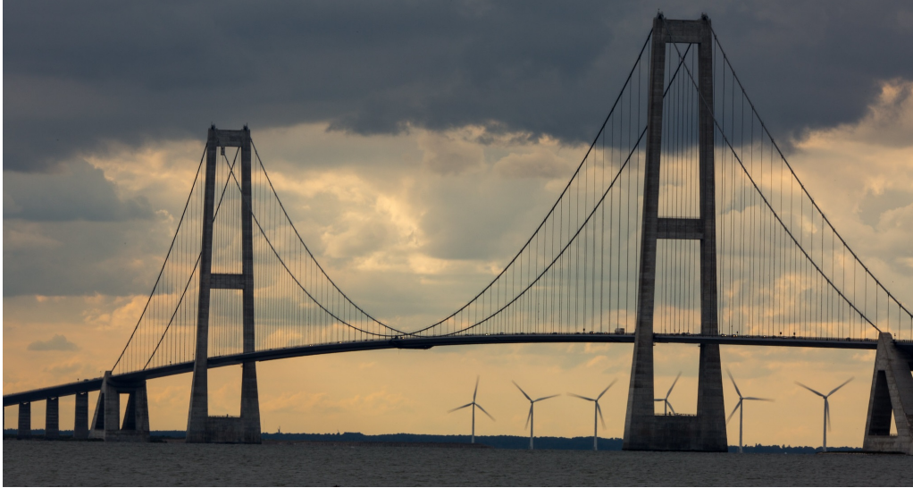
Figure 3.7: Great Belt Bridge. Built in 1998. [29]
