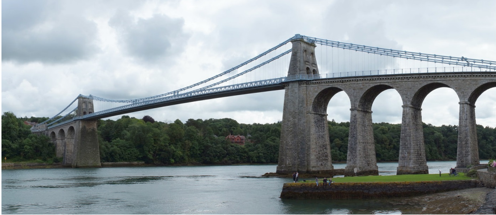
Figure 3.1: Menai Suspension Bridge. Built in 1826. [31]
