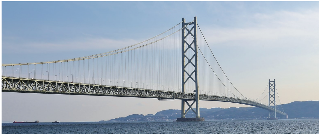
Figure 3.6: Akashi Kaikyo. The world's longest span. Built in 1998. [15]
