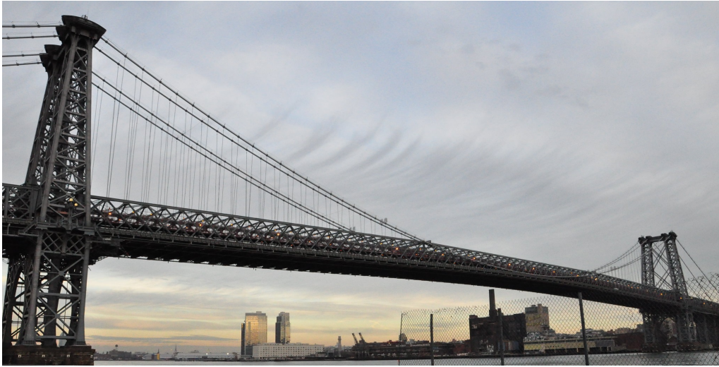
Figure 3.3: Williamsburg Bridge. Built in 1903. [42]
