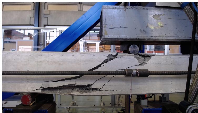
Figure D.15: Shear crack in B6 after the second peak in the load - displacement graph.
