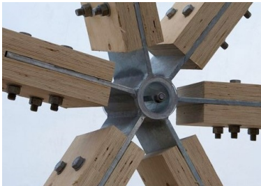
(a) Dome of visions 1.0 in Copenhagen, Denmark. The splices are inserted vertically and welded to a hollow cylinder. Photo: Paul Nybo Andersen (Dome of Visions, 2013)
