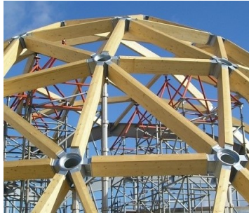
(b) Connectors at the Pods Sports Academy. Here the steel forms a hollow cylinder to where members meet. Photo: Westmuckett Hawkes Ltd (2010)
