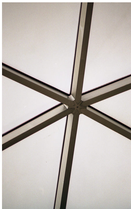
(b) Connector detail of connected steel elements. Photo: Piergiorgio Rossi (2005)
