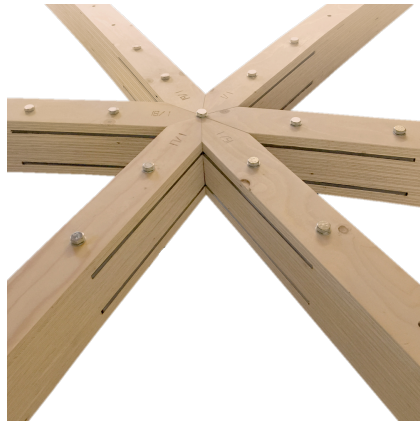
Figure 3.1: Connector design for weight calculations, (Dome of visions, 2017)
