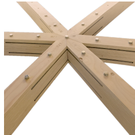
(b) Dome of visions 3.0 in Aarhus, Denmark. The splices are inserted horizontally to the timber elements. Photo: Kristoffer Tejlgaard (Dome of visions, 2017)
