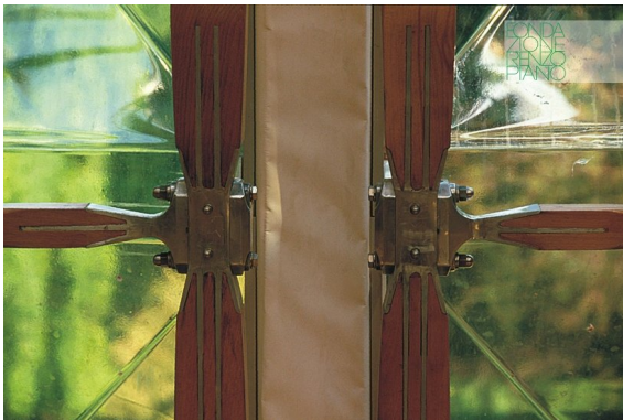
(a) Timber-aluminium joint in IBM Travelling Pavilion, Photo: ©Gianno Berengo Gardin (Fondazione Renzo Piano, n.d.)
