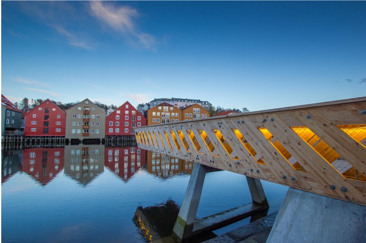
Figure 2.2: The Trondheim HolzBau Pier (2014). Architects: John Haddal Mork and Anders Gunleiksrud. Photo: Sophie Labonnote-Weber [2]
