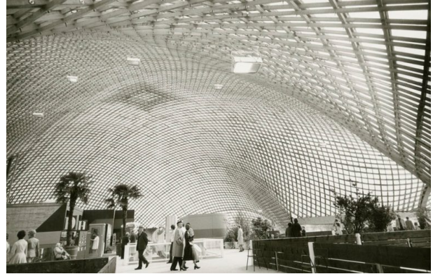
(b) Inside Mannheim Multihalle.
