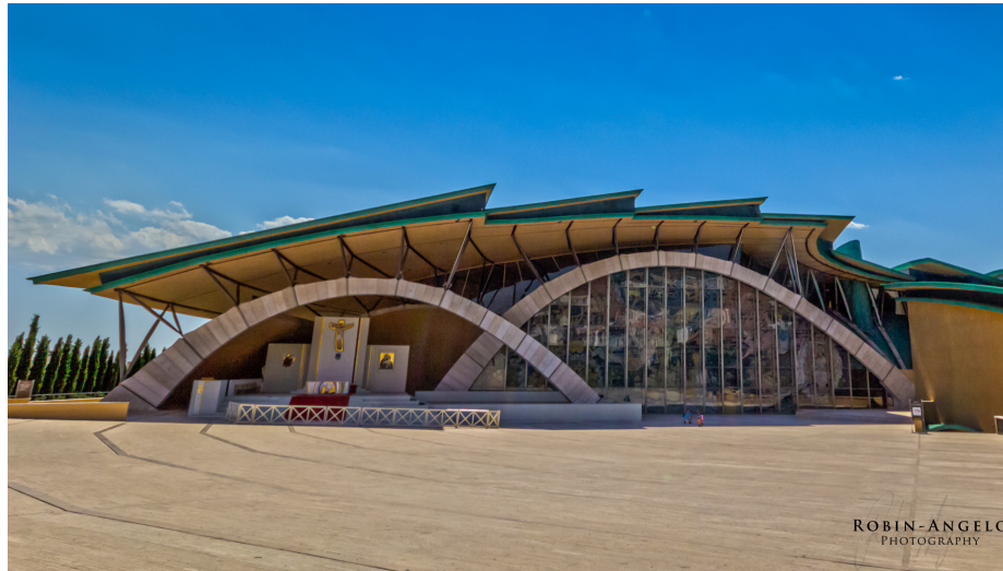
Figure 3.11: The Church of Padre Pio. The whole building consists of a series of stone arches arranged in two half-circles around a centre point. Image from: Robin-Angelo (2012).
