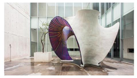
Figure 1-4: KnittCandela, an ultra-thin concrete shell by researchers at ETH Zürich [5].
