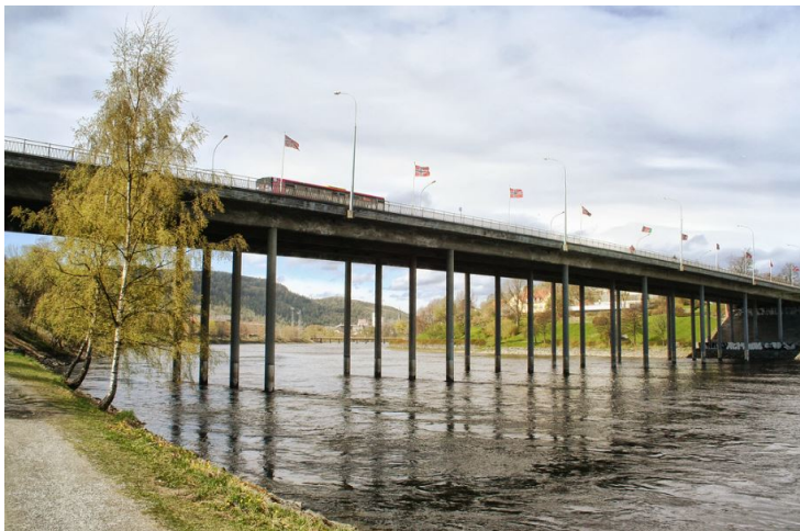
Figure 4.1: Overview of Elgeseter bridge seen from the west [28]
