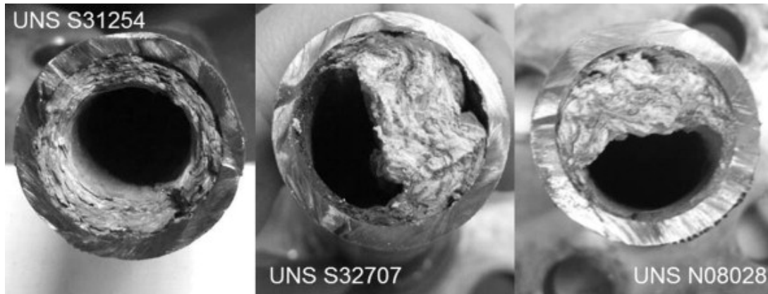
Figure 1.2: Cross-section of stainless steel pipes: (left) partially clogged straight pipe, (middle, right) partially clogged outlet of bends. The figure is taken from Karlsdottir et al. (2014).
