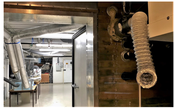
Figure 5.2: Sniffing port connected to the supply air outlet.
