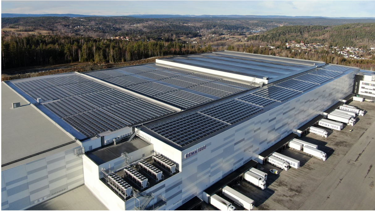
Figure 1.6: Login Vinterbro with PV system installed [17].
