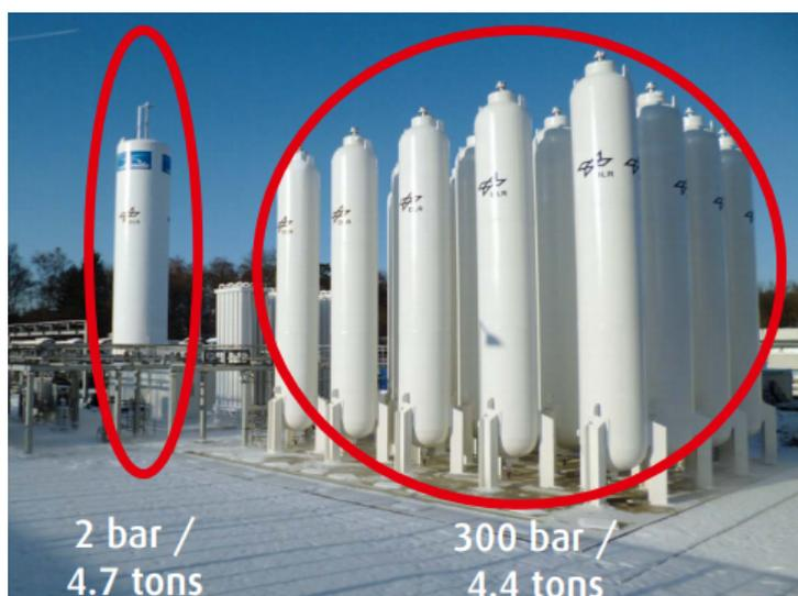
Figure 2.12: Illustration of Liquid and compressed hydrogen storage tanks [77].
