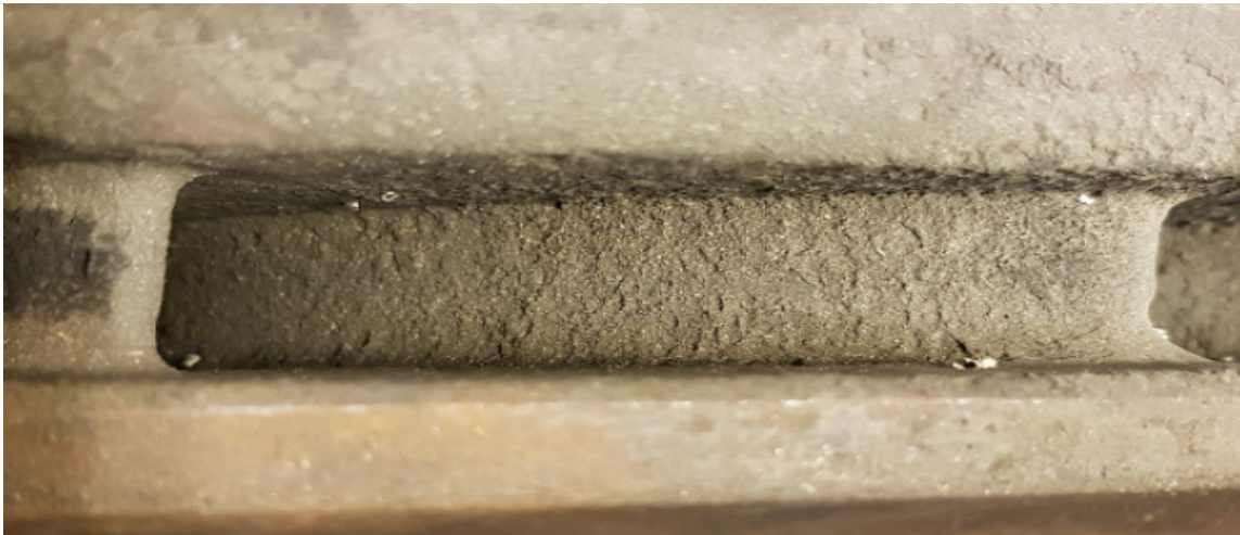
Figure 11: Fouled impeller of a compressor, NTNU Test Facility.
