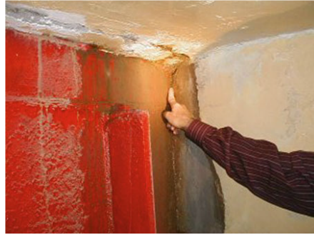
Figure 2.5: Damage caused by Vortex rope [4]
