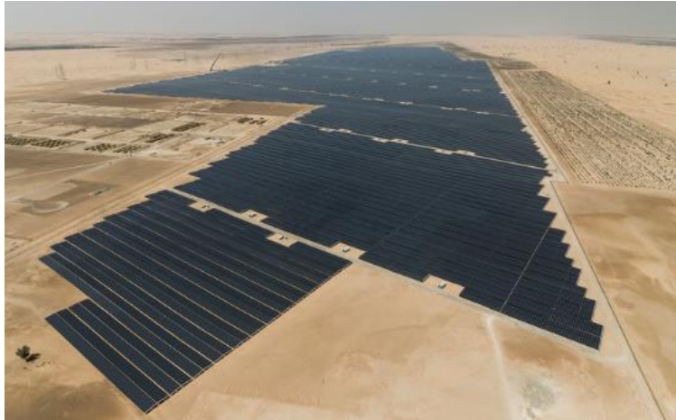
Figure 2.6 Sweihan solar plant [22]
