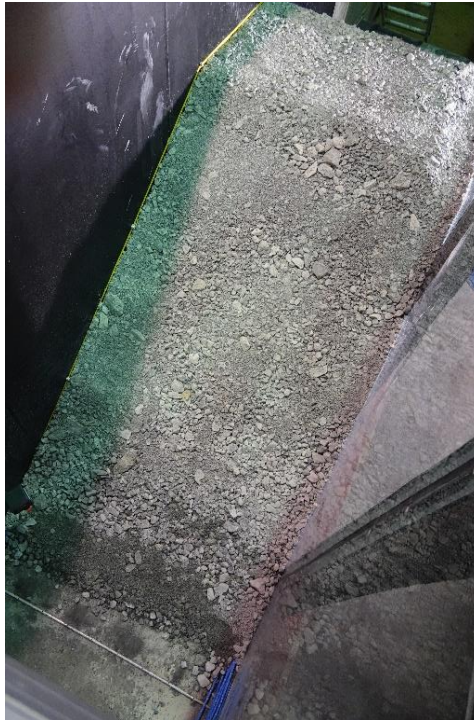
Figure 25 End of construction
