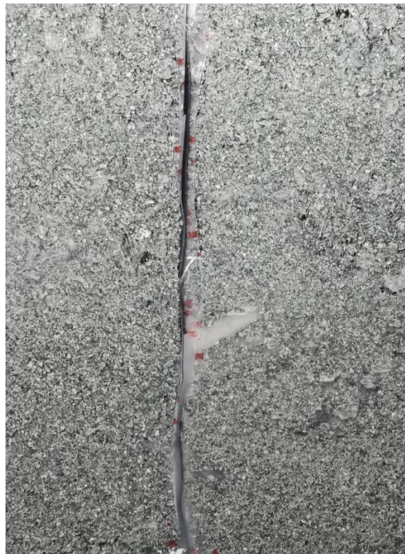
Figure 28 Watertight core plastering to flume
