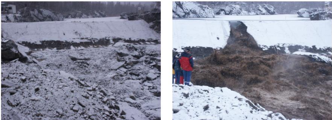
Figure 17 Initial erosion in pilot channel and (b) breach enlargement during dam breach field test in Norway (EBL 2003)
