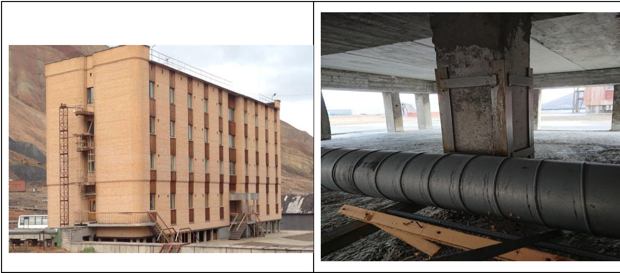
Figure 4-1 Building supported by concrete piles in Pyramiden, Svalbard, Norway
