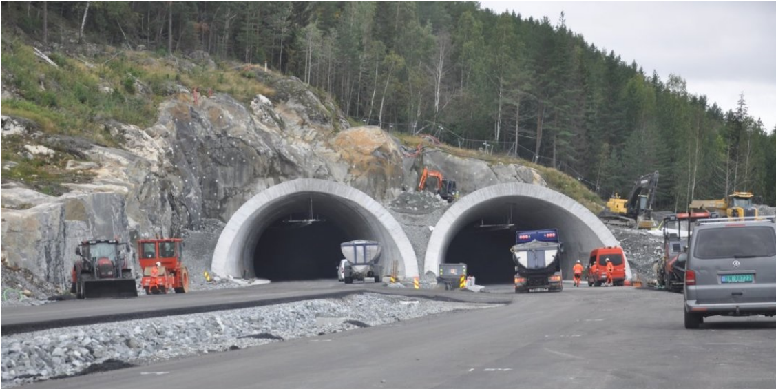
Figure 11.2: The Svartås-tunnel under construction, September 2019 (Kjell Wold 2019)
