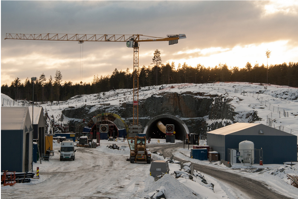
Figure 12.2: The Kongsberg-tunnel under construction, March 2017 (Unlisted 2017 )
