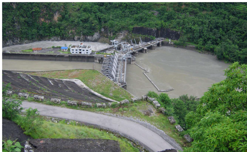
Figure 4.1: Existing headworks of KGA during wet season operation (Biswhwakarma, 2018).
