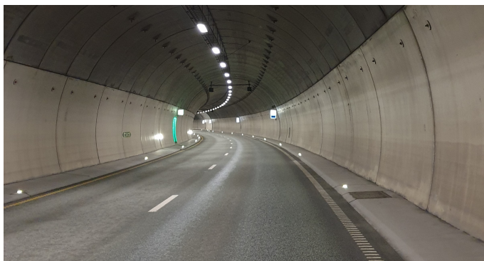
(a) Tunnelhvelving, Strindheimtunnelen
