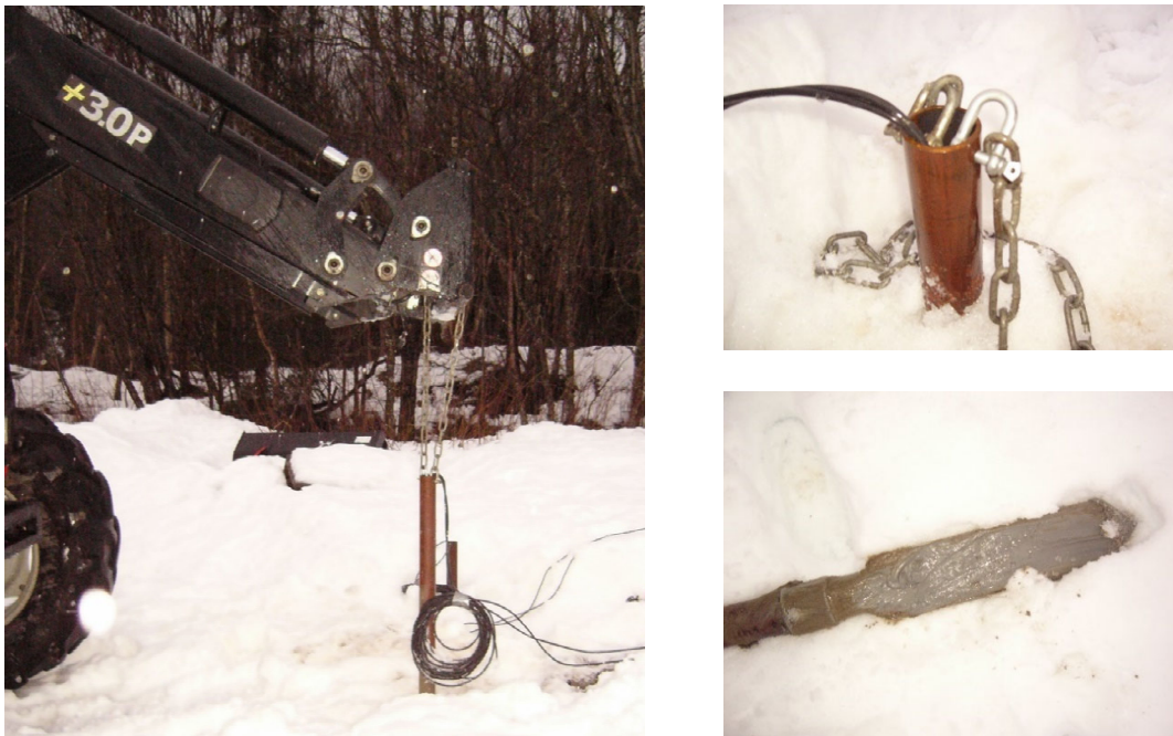
Figure 4- 2 Cell extraction procedure for first installation at 5 m
