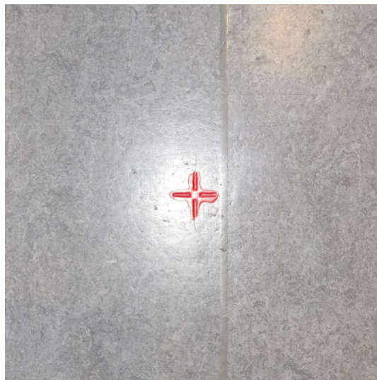
Figure 3.1: Example of benchmark on linoleum floor
