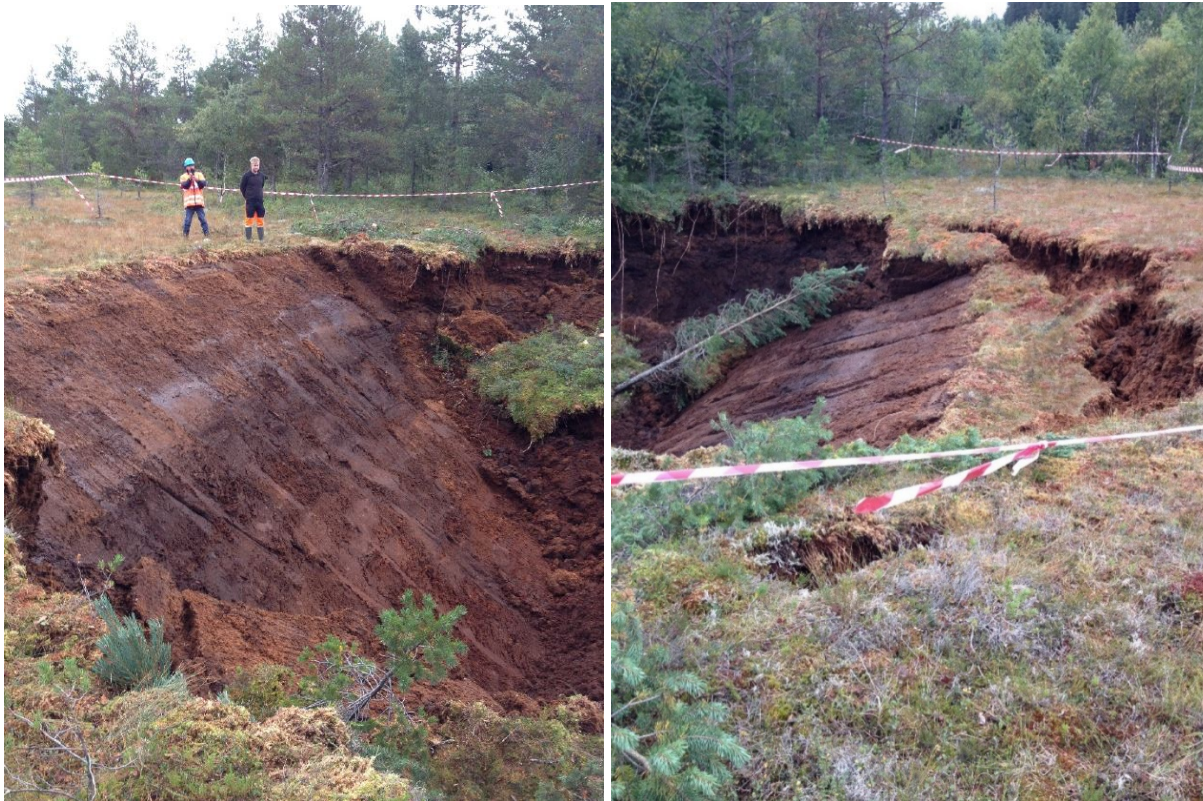
Figure 20 Failure at a peat excavation at Tanemsmyra, near Trondheim.
