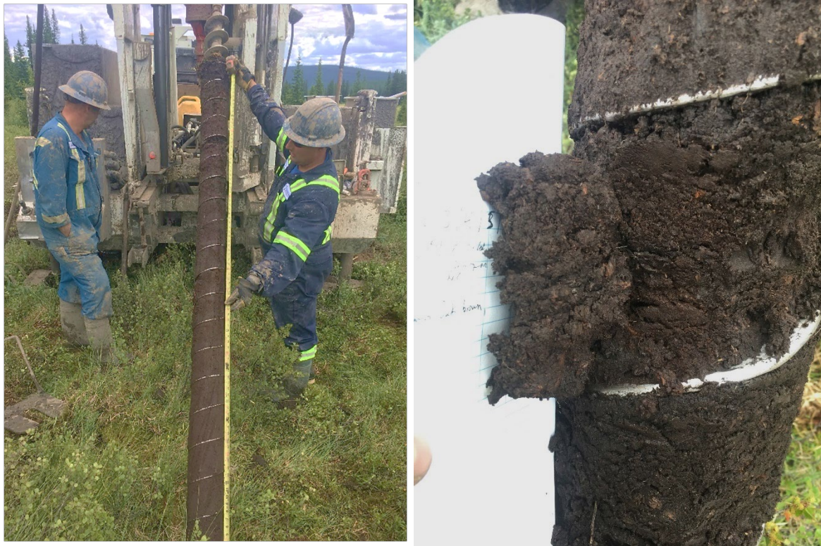
Figure 3 (L) Peat exploration near Hinton, AB, Canada. An auger drill rig recovers 3 m of peat, while positioned on a swamp. The auger rig is placed on wooden plyboards for stability. (R) A close-up of the peat sampled. Fibres and plant material can be observed (Photos take by Omar Berbar).
