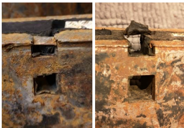
Figure 4.11: Damaged mounting holes, from blades worn down too far
