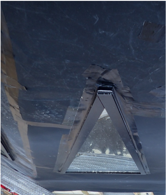
Figure 2: Tape used to seal the wind barrier around a window.
