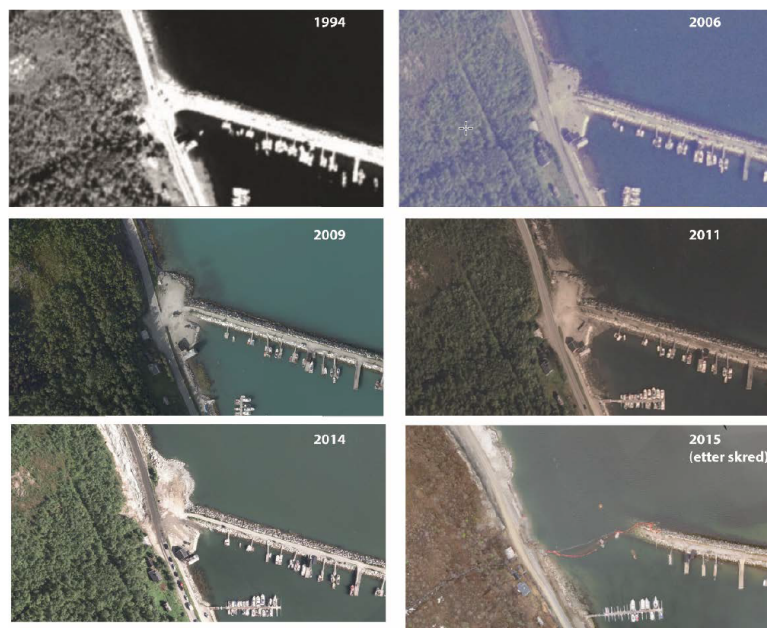
Figure 7.29: Pictures of the breakwater construction stages from 1994 to 2014, and the post-slide image from 2015 where the breakwater has collapsed, retrieved from (Nordal et al., 2016).
