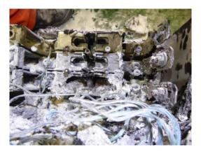
Figure 1-1: Arc flash in a contactor, courtesy of BW Offshore.
