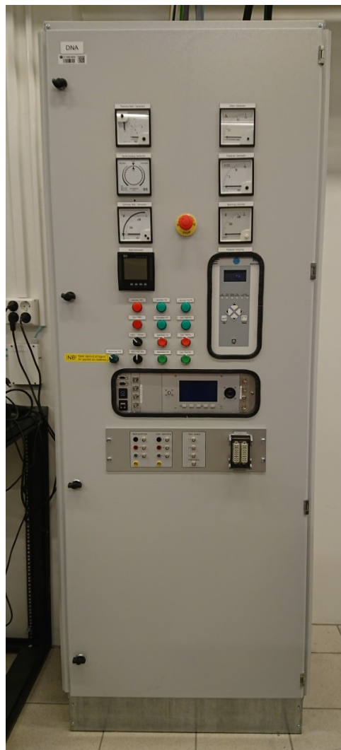
Figure D.1: Picture of the control cabinet for the Siemens-Schuckert motor/generator set.
