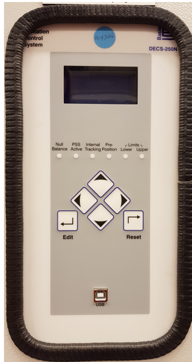
Figure 3.5: Control panel for the Basler Electric DECS-250N digital excitation control system.
