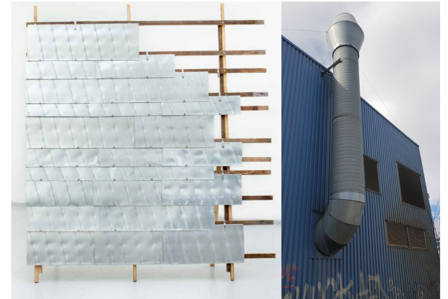
Figure 14: Reused ventilation ducts as cladding.
