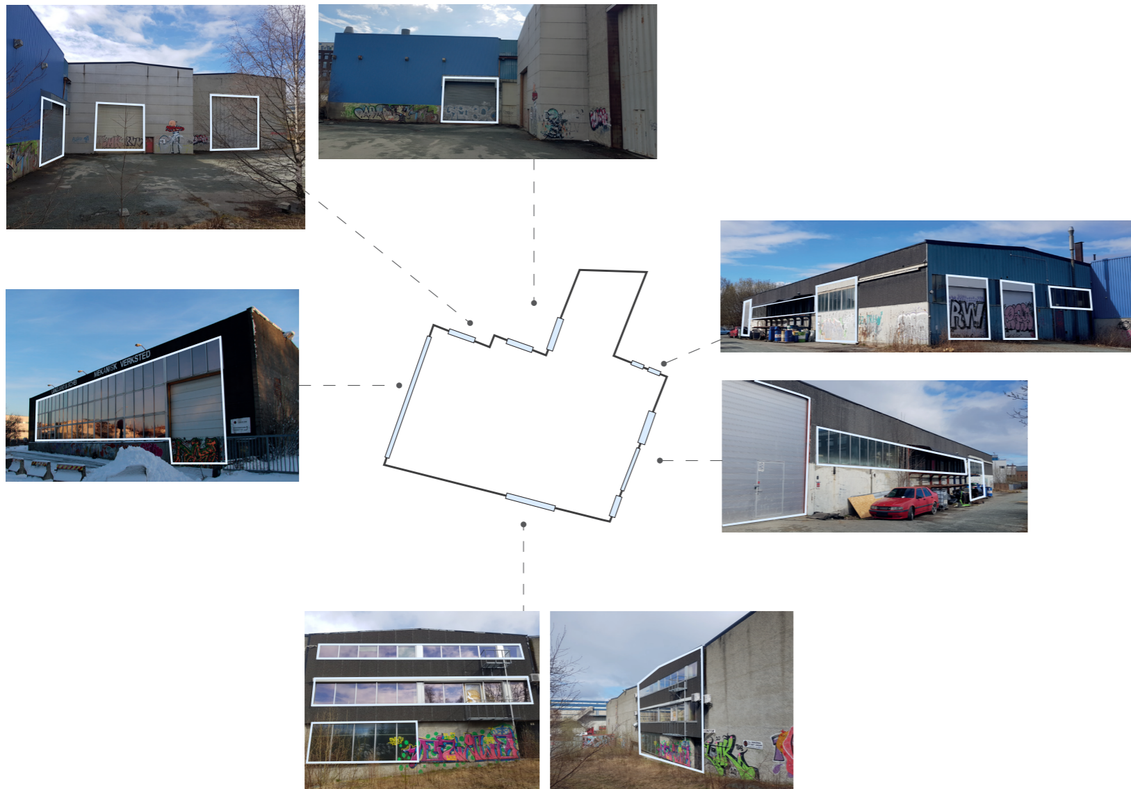
Figure 43: Map of existing openings in the facade.
