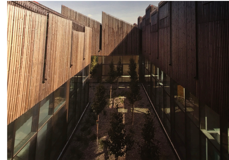
Fig. 18. View of an interior courtyard that provides daylight, natural ventilation, and views to the garden. Floor-to-ceiling glazing complements the toplighting and stack ventilation from the skylights. Direct sunlight and heat gain can be mediated by interior shades.
