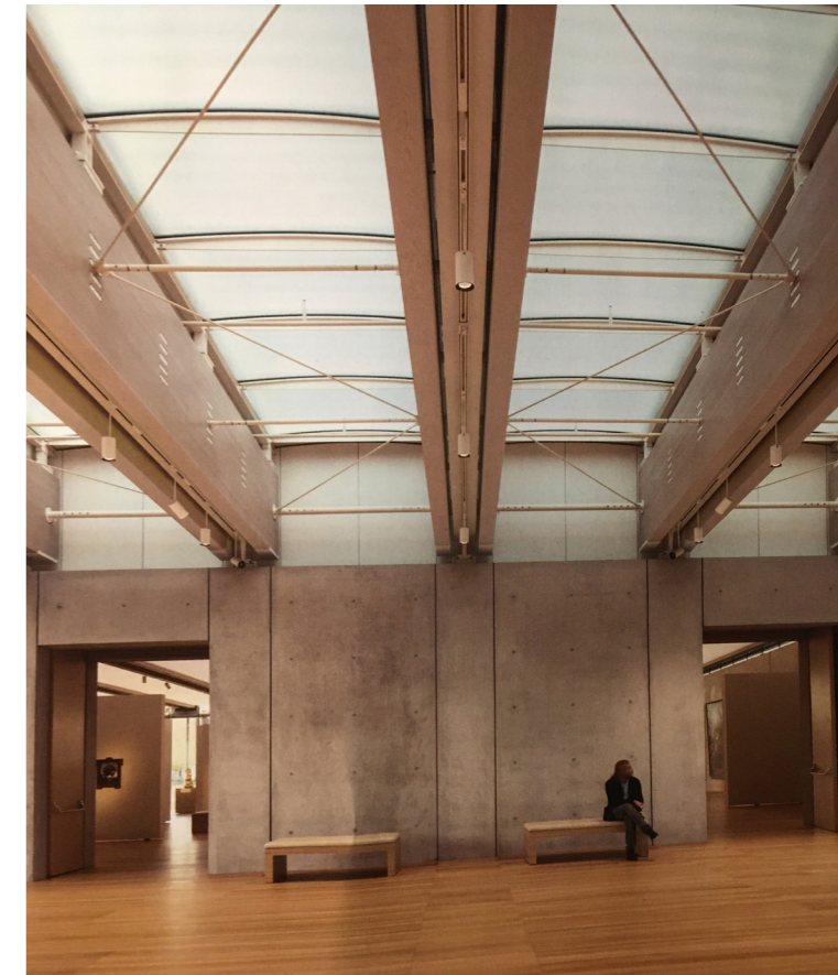
Fig. 22. Expansive translucent skylights with exterior shading louvers capture north light and provide an even distribution of daylight in the entry lobby. Piano Pavilion, Kimbell Art Museum, Fort Worth, Texas, USA; Renzo Piano, Renzo Piano Building Workshop.
