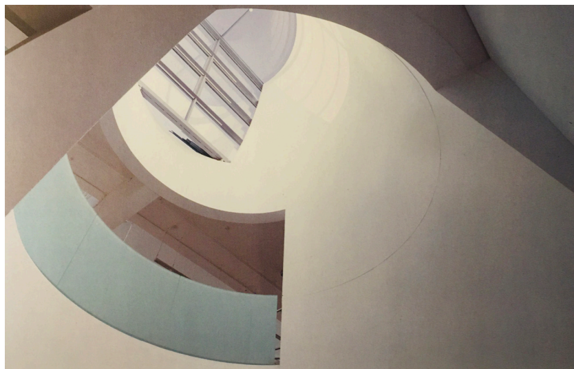
Fig.16. Detail of a 'driven void of light' reveals the large south-facing skylight with operable windows that admit light and exhaust air.
