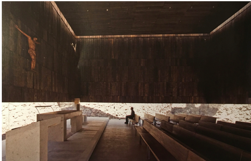
Fig. 19. Structural loads of the chapel are carried to exterior piers in the rock walls of the garden. From the interior, the rustic wood volume appears suspended inside the structural glass curtain wall. Sunlight reflected off the stone walls into the lower portion of the chapel through the glass facades is complemented by a soft band of daylight from a narrow skylight at the top of the chapel.
