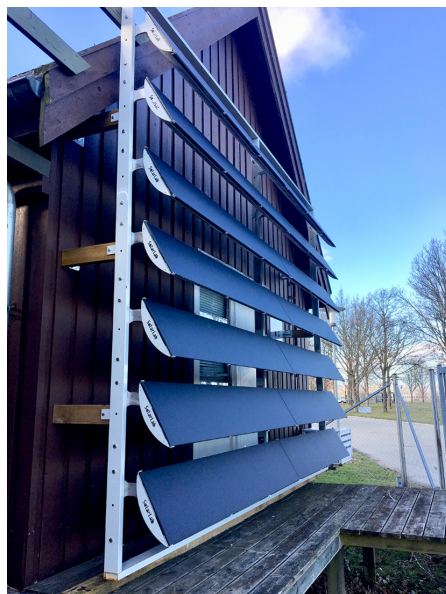
Fig. 1. A PVSD product from SOLARLAB at the BIPV demo site of the Danish Technological Institute in Høje-Taastrup (Denmark).
