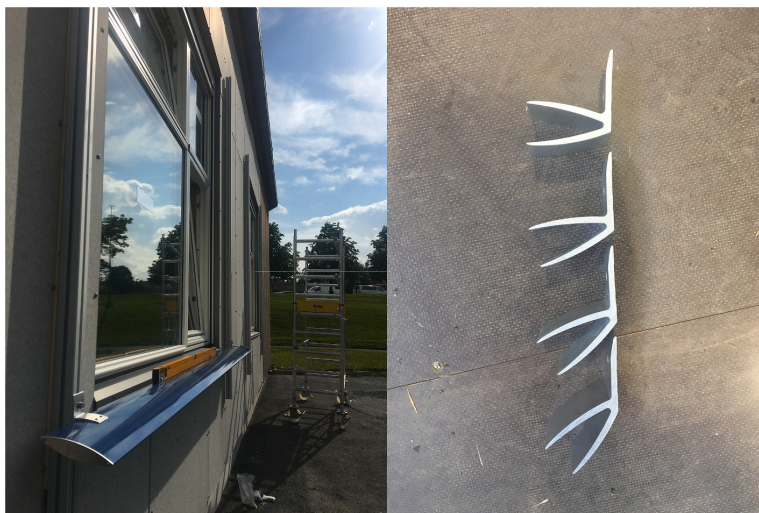
Fig. 1. Attachment of a blue louvre (left) and brackets for the four different angles the louvres can be tilted at (0, 15, 30, and 45° from horizontal) (right).
