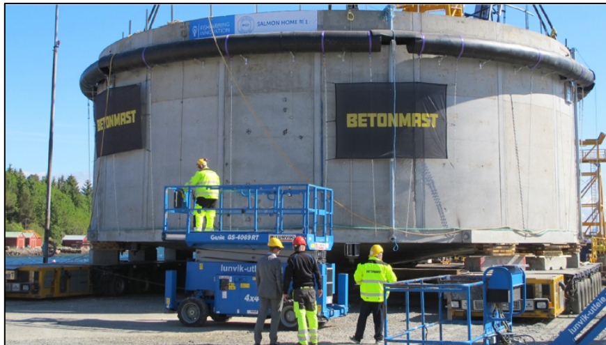
Figure 27a: Concrete containment fish tank (Picture courtesy of Tor Ole Olsen)
