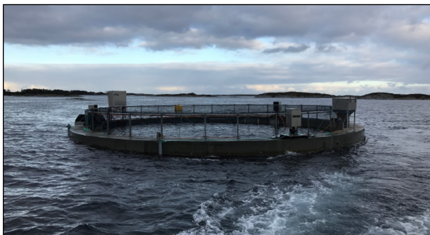
Figure 27b: Concrete containment fish tank on site (Picture courtesy of Tor Ole Olsen)
