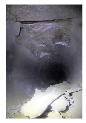
Figure 16. Example of block fall witnessed in Ulset headrace tunnel in 2017.
