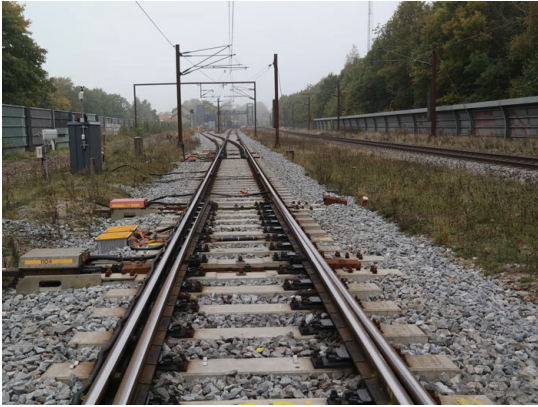
(a) Beginning of the railway turnout
