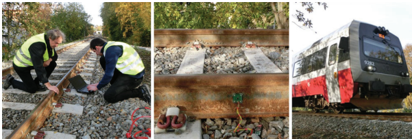
(b) Installation of the sensor
