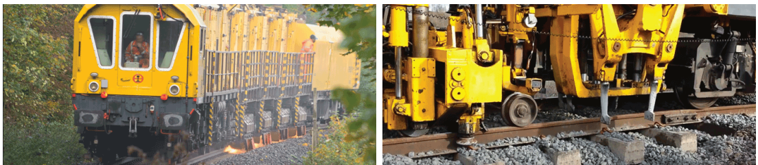
(a) Rail grinding
