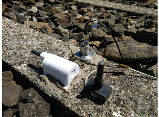
(b) Railway sleeper location
