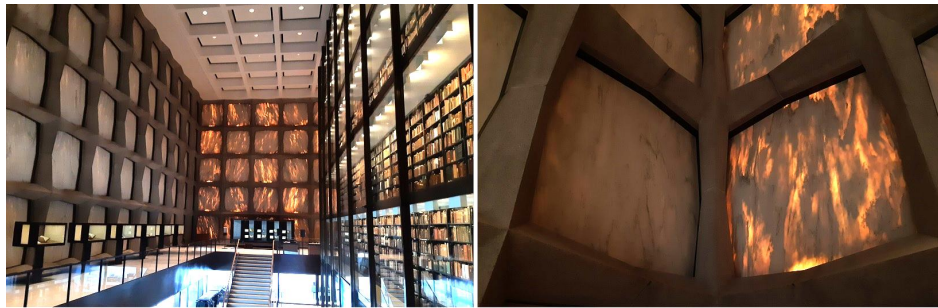
Figure 1.1: Beinecke Rare Book and Manuscript Library is located on Yale University campus, in New Haven, Connecticut. It was designed by Gordon Bunshaft and the construction was completed in 1963. The library is built with translucent marble panels. This is a vivid example of using translucent building materials in modern architecture and respective visual appearance generated with that. While the panels look opaque most of the time (the left wall in the image), they start to transluce and glow (the right wall) as soon as direct sunlight hits them. The visual effect is achieved with a phenomenon that objects look more translucent when they are back-lit. [Photo by Davit Gigilashvili]
