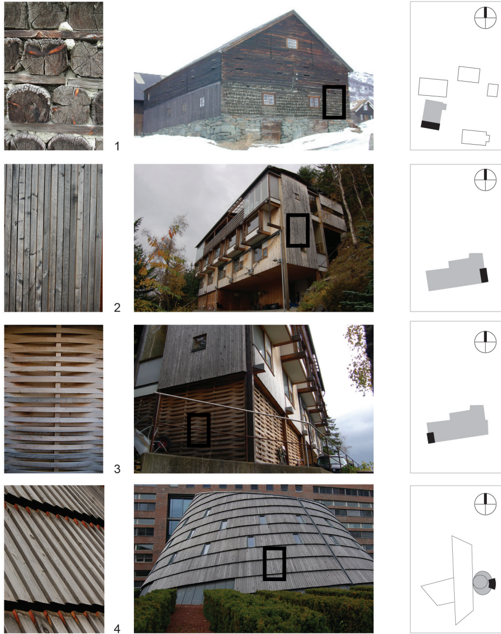
Figure 1.1 Examples of weathered untreated wooden façades. 1: Stovewood barn. Ner Skjørtad, Oppdal, Norway. Construction year around 1840. Photo taken 2004. 2 and 3: Villa Kittilsen, Ålesund, Norway. Architects: Jensen and Skodvin. Construction year 1997. Fotos taken 2007. 4: Hamar town hall, Hamar, Norway. Architects: Snøhetta. Construction year 2000. Photo taken 2007.
